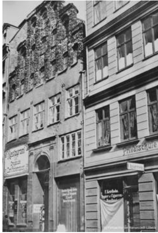
The original buildings at Königstraße 93 and 95.
