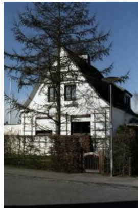
The house at Neuer Faulenhoop 22 in Lübeck-Karlshof; photograph: Heidemarie Kugler-Weimann, 2008
